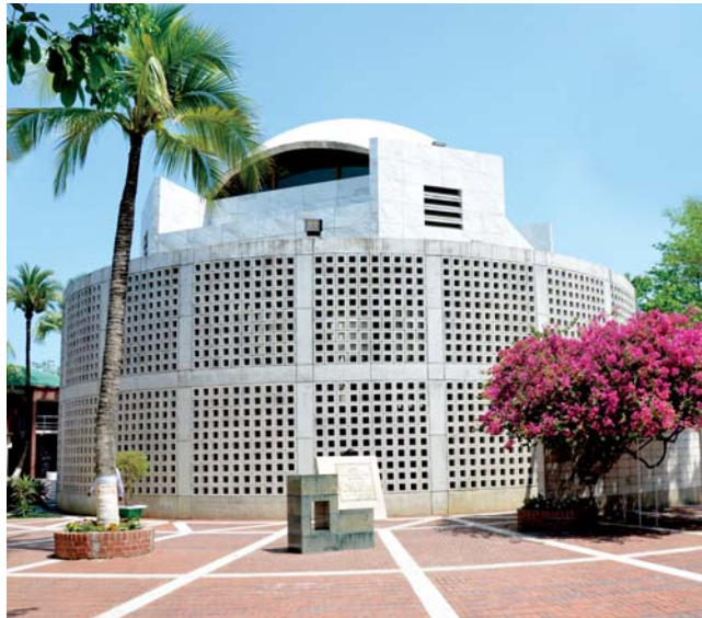
Bangabandhu Mausoleum Complex, Tungipara, Gopalganj
